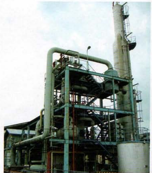
Resin plant undergoing refurbishment
